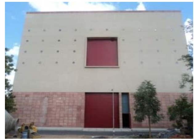
ITER-India Lab Building
